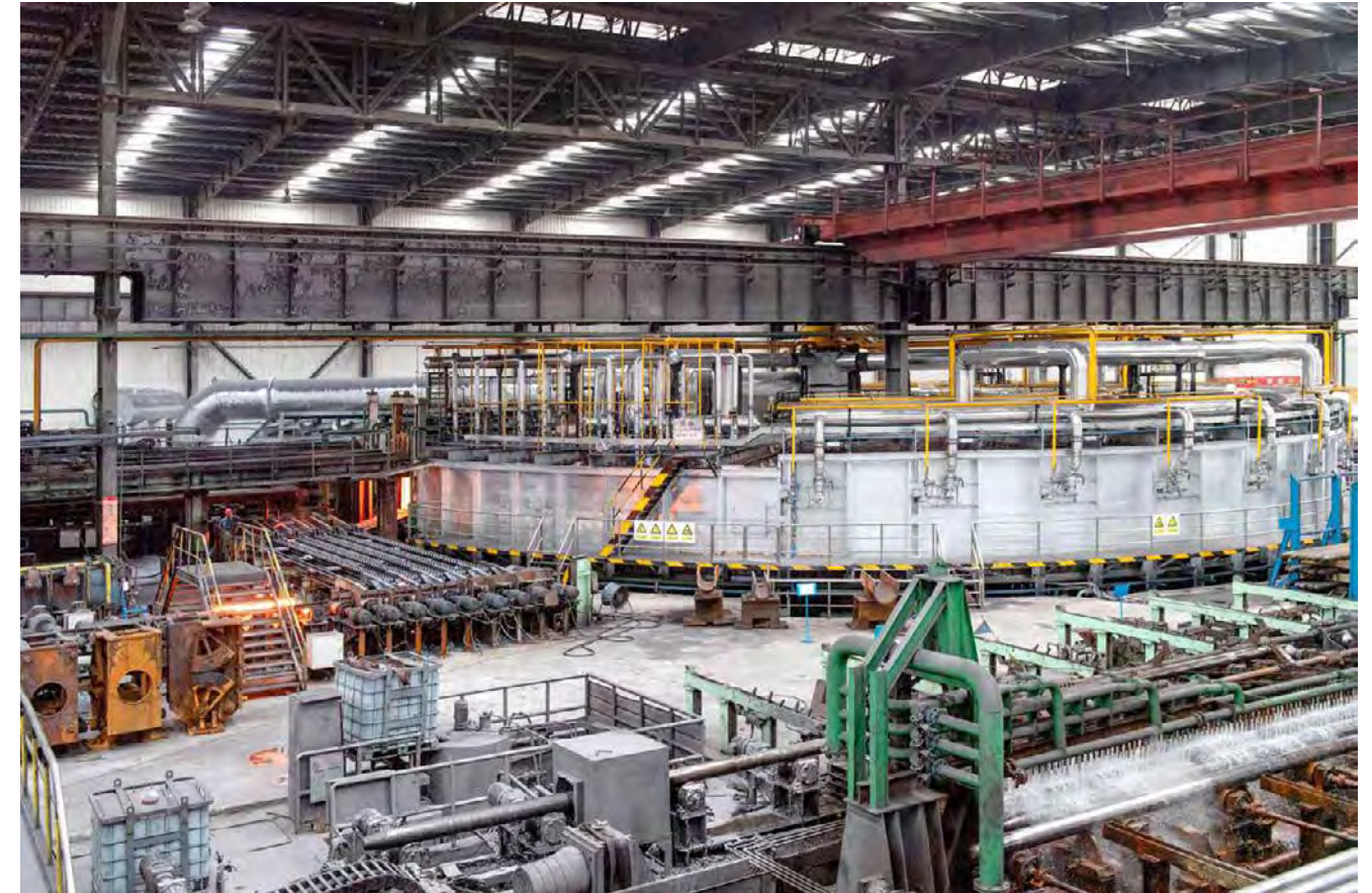
★ Ring heating furnace
